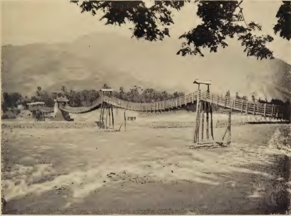
BAMBOO SUSPENSION BRIDGE, SLUNG ON BAMBOO ROPES, AND ABOUT 700 FEET LONG
